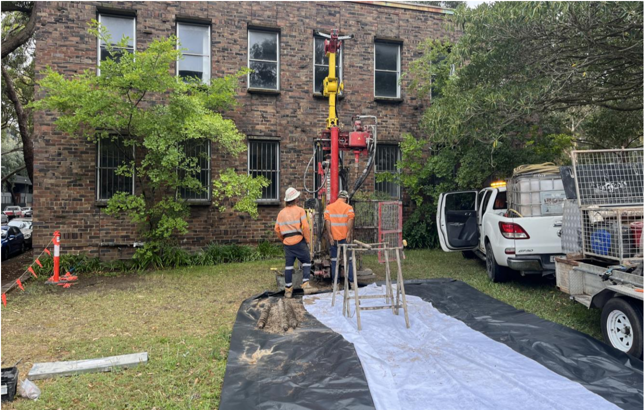
Figure 2-Photo of the drilling setup.
